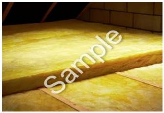
Insulation should be installed tight to the structure, without air gaps, and should extend to the wall insulation.
