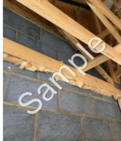
Eaves photograph should show loft insulation extending beyond the wall insulation to minimis cold bridging.
