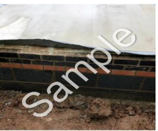
Moisture-resistant insulation should be fitted below damp-proof course level and extend to the foundation block/structure.
